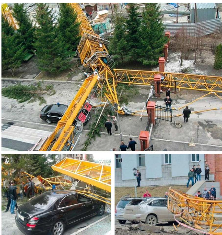
Fig. 59. Fall of a crane on construction site of an apartment house in Novosibirsk: a — general view of tower crane QTZ-80; b, c — damaging cars parked near by
