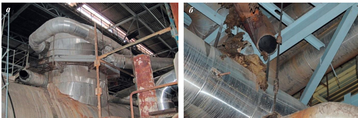
Figure 30, a, b. The area of destruction of the heating steam pipeline of Unit 2 at the branch of Thermal Plant of Samara of JSC Volzhskaya TGK
