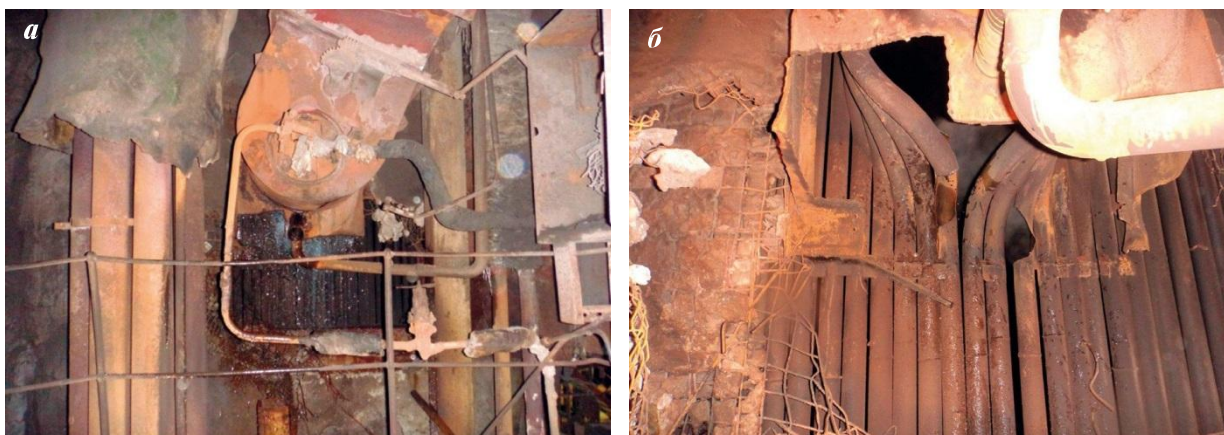
Figure 32, a, b. The view of the area with the rupture of wall tubes under the fuel nozzle of the left wall of BKZ-210-140-8 boiler.
