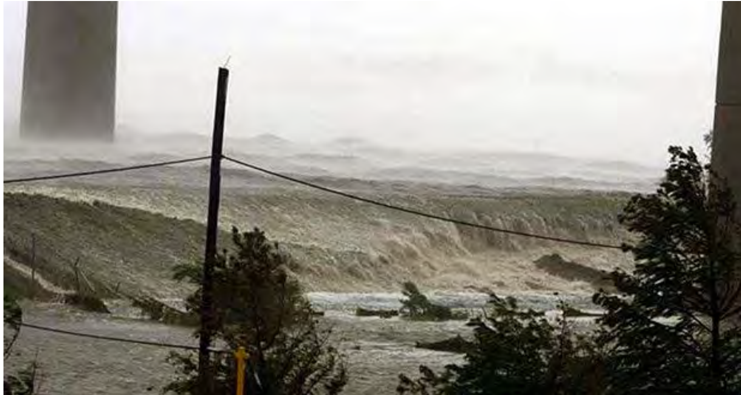
Mississippi River Gulf Outlet (MRGO) Levee Over-topping
