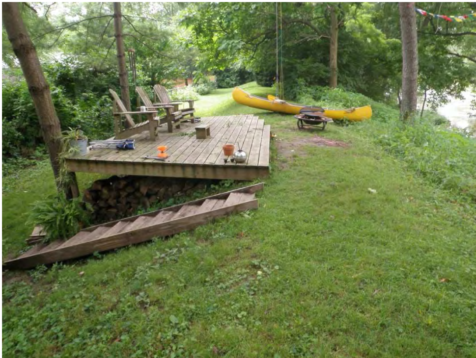
Photo 40: Deck encroaching onto levee (looking southwest near Station 77+80)
