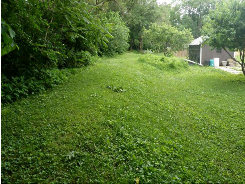
Photo 39: Levee embankment (looking east near Station 72+50) Note the dense vegetative growth on the riverward slope.
