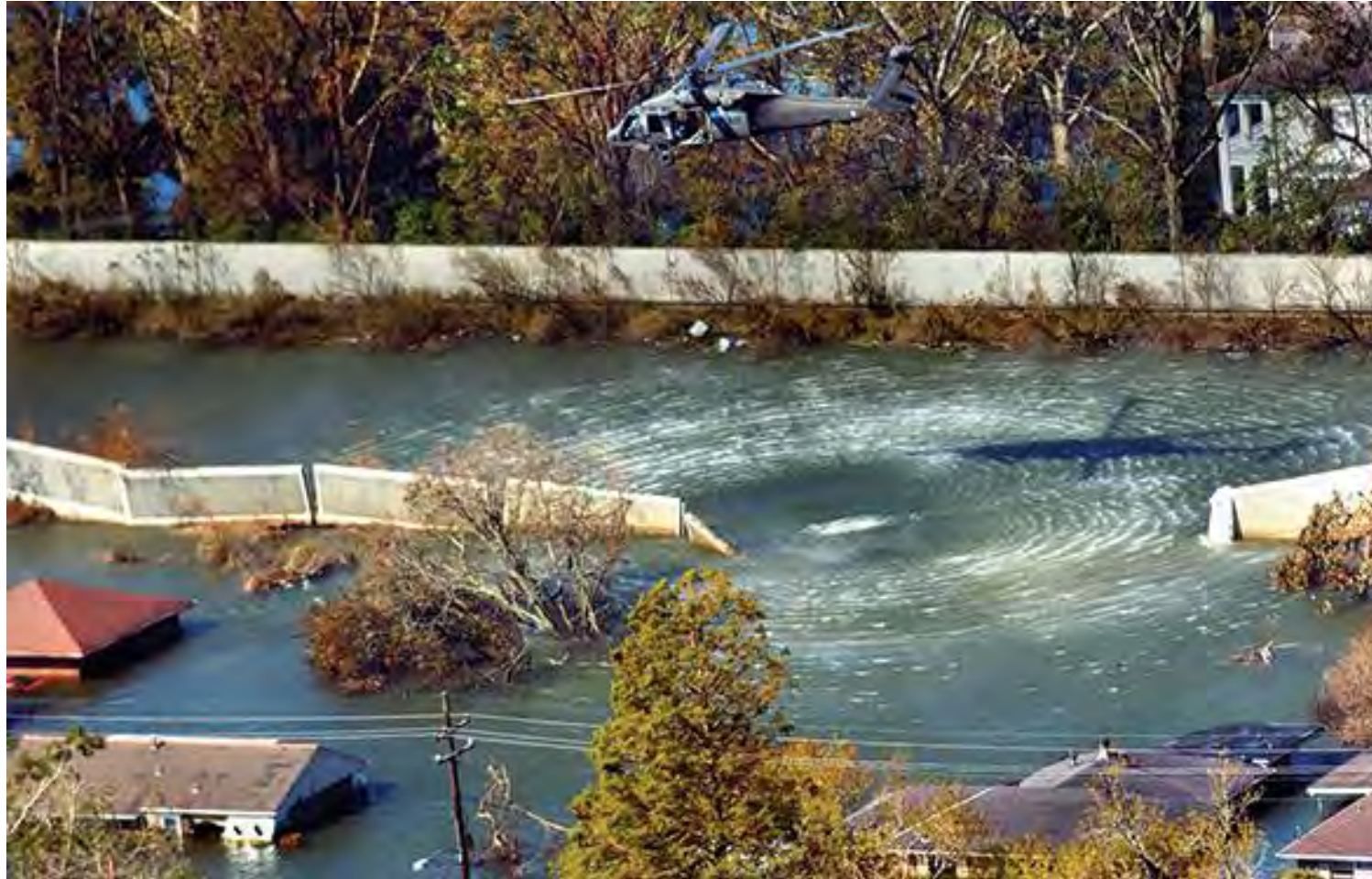
London Avenue Canal T-Wall Breach
