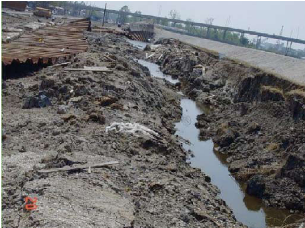
Figure 7.9 Industrial Canal East Bank South Failed I-wall
