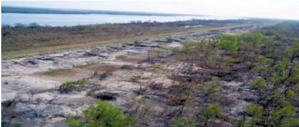
Figure 7.12 Obliterated Levee along the Mississippi River-Gulf Outlet
